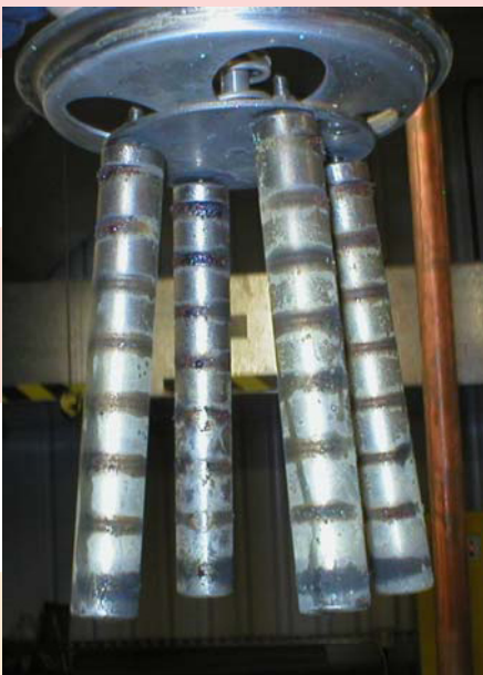
Magnets in a clean water circuit
